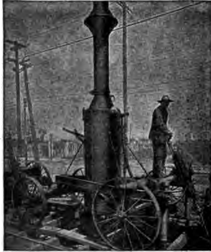
Fig. 167. Portable Boiler and Drill for Trench Work.
